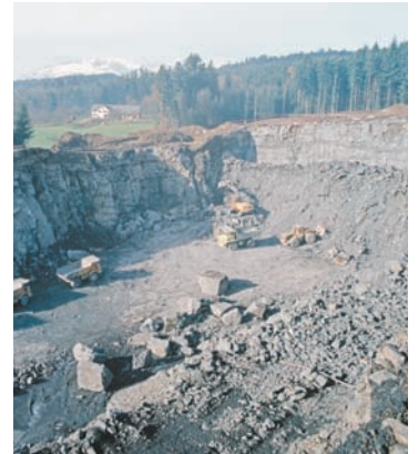
Baugrube Ambergtunnel, November 1979
